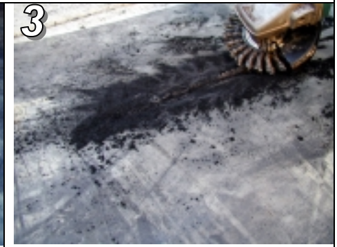
3 The blade will leave a smooth shiny finish so the rubber needs to be or roughened to improve the bonding properties. Use a wire brush on the slowest grinder setting
